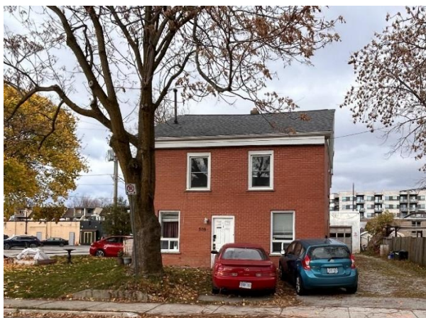
Figure 2 – Front façade (south elevation)
