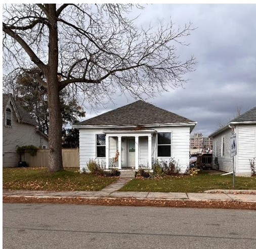
Figure 14 – Front façade (south elevation)
