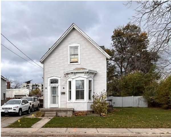
Figure 6 – Front façade (south elevation)
