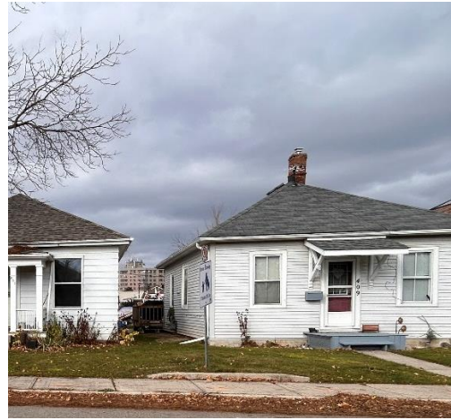
Figure 18 – side façade (south-west elevation)
